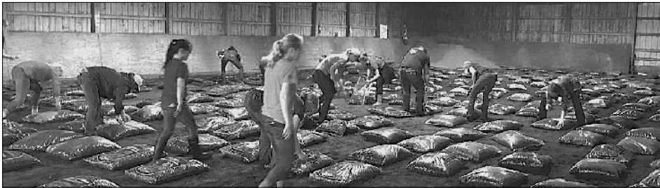
Cedarville University students spreading new rubber footing around the indoor arena.
